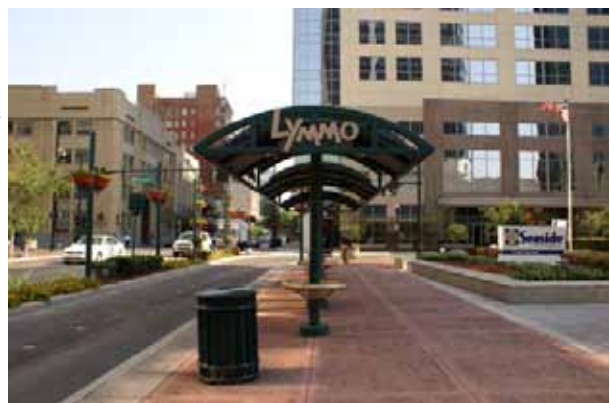
A separate traffic lane is reserved for the LYMMO circulator bus in downtown Orlando.
