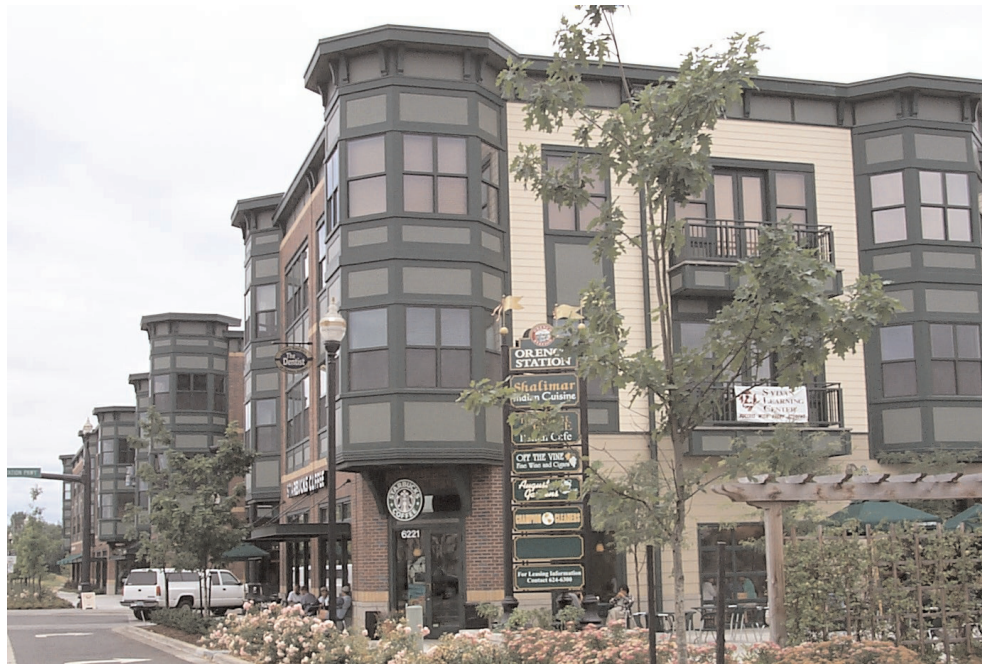
Orengo Station, along TriMet’s Westside MAX Blue Line, is a 200-acre transit-oriented development featuring retail, commercial, and housing. The buildings shown here in Hillsboro feature mixed-use retail and housing. The Orengo Station Community was voted the Best Planned Community by the National Association of Home Builders in 1999.
