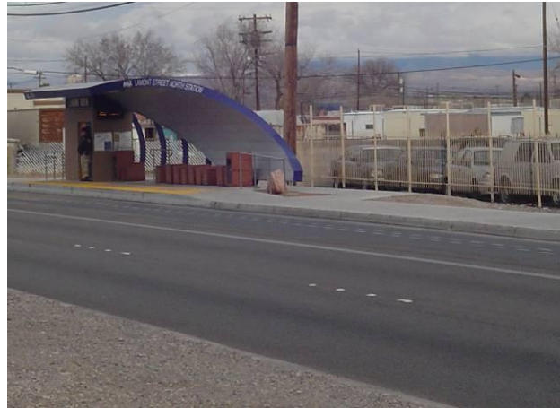
Figure 4. Original Station Design with Fence Blocking Pedestrian Access
