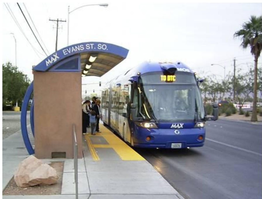
Figure 1. Running Way, Vehicle, and New Station
